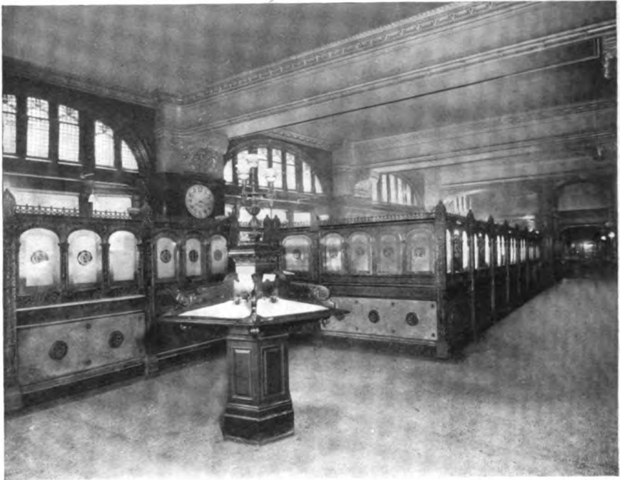
MAIN BANKING ROOM
